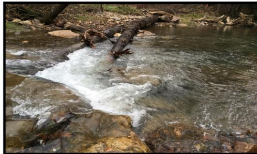
*A newly constructed log and rock cross vane, in the South Fork of Bens Creek mitigation site*
