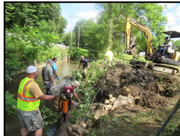
The funding combined with in-kind contributions from the Conemaugh Township Supervisors, enabled the stabilization of the streambank and created habitat for the trout with the construction and placing of log vanes, muddills, root wads, j-hooks and random boulders.
