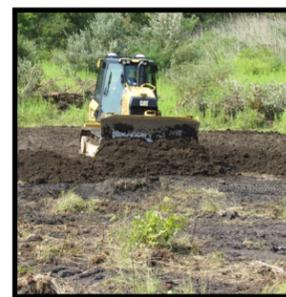
*Topsoil being spread during the Revegetation Project at Hawk View.*
