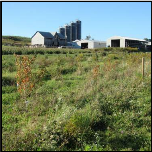
A section of the completed stream buffer.
