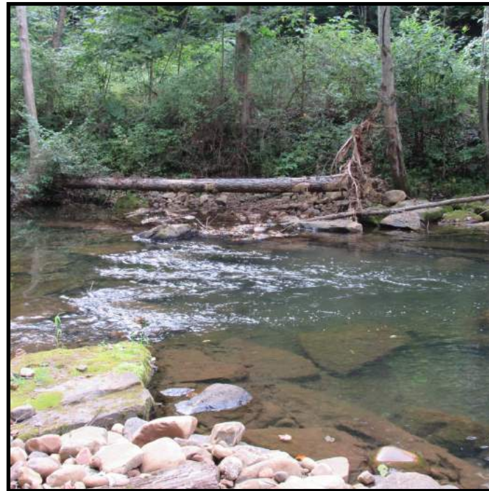
Rock and wood placement along with bank stabilization on the Que Tailwater.
