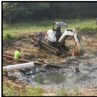
Sludge is removed from Oven Run AMD Treatment System Site F (Hawk View) as a part of the District's perpetual responsibility for operation and maintenance of the Oven Run treatment systems on the Stonycreek River.
